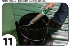
Seal the adjusting seam and the base/elbow connection seam on the inside with roofing cement. Seal locking clamp holes and all
