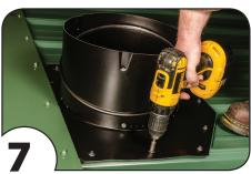
Secure to the roofing metal with sheet metal screws at the top, sides, and bottom.
