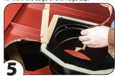
Using 1" wide butyl tape, seal around the base flashing. Position tape to ensure good roof. Remove any roofing screws as necessary. compression and weather tight seal to roof
