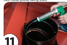
cement. Seal locking clamp holes and all exposed screws with roofing cement.
