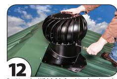
Position the Whirlybird turbine head on the base. Line up the predrilled holes in the brackets and elbow and fasten with sheet metal screws.
