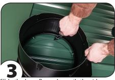
Slide the base flange beneath the ridge cap indicator line on the base flashing. Place 3 ensuring ridge cap completely covers the base flange. Locate base opening between
