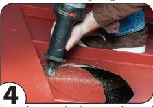
Locate base opening between rafters and mark hole to be cut. Locate rafters by tapping Cut hole as marked. Take care not to let cut metal being used. out fall into the attic space.
