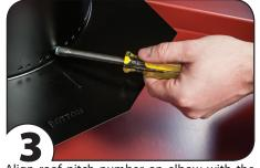
Align roof pitch number on elbow with the indicator line on the base flashing. Place 3 screws through holes that line up with predrilled holes in base
