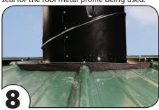
Make certain tape location will ensure good compression and weather tight seal for the roof metal profile being used.
