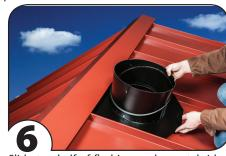
Slide top half of flashing under metal ridge cap while aligning base with cut out. Take care that tape location will ensure good compression and weather tight seal for your roof metal's profile.
