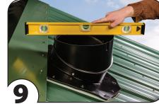
Rotate top of elbow to level position by turning counter clockwise.
