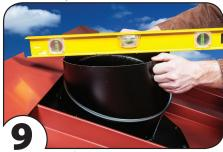
Rotate top of elbow to level position by turning counter clockwise.
