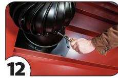
Seal the adjusting seam and the base/elbow Position the Whirlybird turbine head on the connection seam on the inside with roofing base. Line up the predrilled holes in the brackets and elbow and fasten with sheet metal screws.
