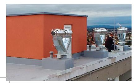
Lomanco sets for flat roofs and sets with electric motor are best placed as an alternative to central electric ventilators in multi-storey buildings such as apartment and tower blocks. The vent turbine sits externally on the top of ventilation shafts to use the wind to remove any unwanted odours from units in a building, with the electric ventilator giving the vent an extra boost if there are poor weather conditions or the tenants choose to open the vents.
