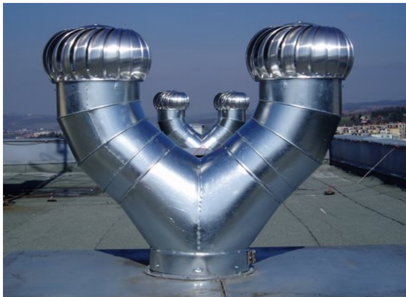
Wind turbines with splitter on a ventilation shaft in block of flats
